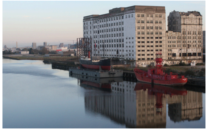
View of Spillers Millennium Mills, Royal Victoria, 2023.
