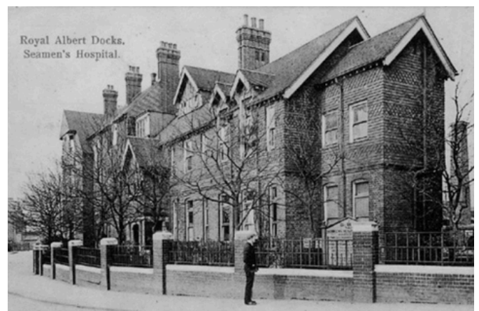
Image: Royal Albert Docks, Seaman's Hospital Location: Alnwick Road, Custom House, E16 3EZ.
