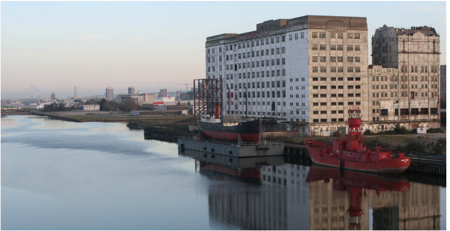
View of Spillers Millennium Mills, Royal Victoria, 2023.
