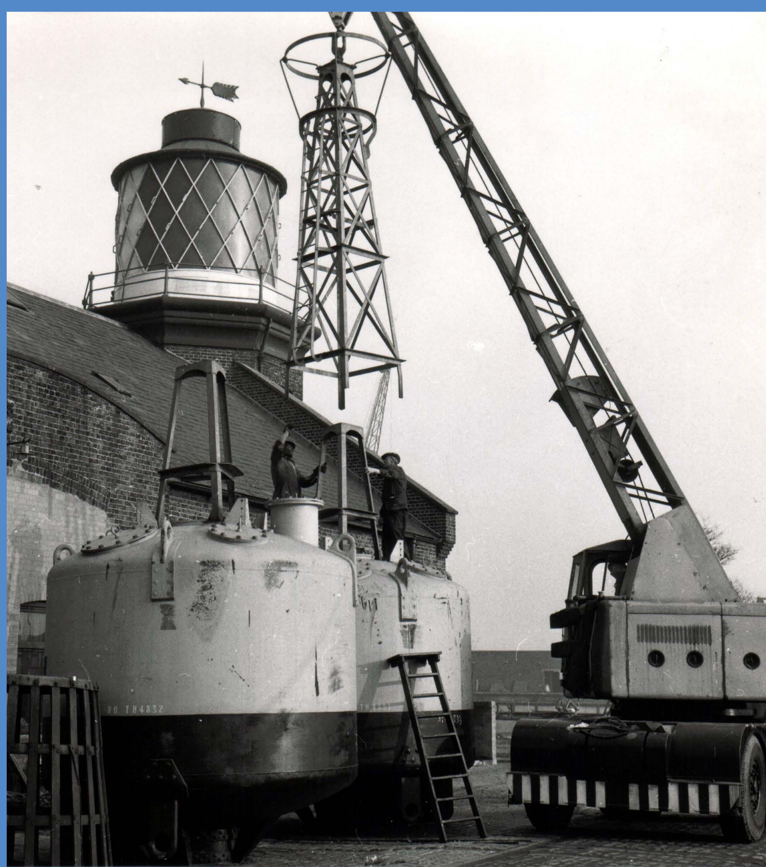
Above left: Lifting a lantern supporting trestle onto a high focal plane buoy, 1959. Trinity Buoy Wharf
